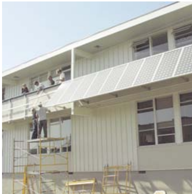
The installation crew mounts photovoltaic panels on the second floor balcony.
