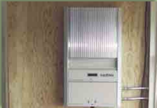
The Xantrex GT3 series inverter assembly complete (above), and with the inverter removed, leaving the handy wiring box (shown open, at right).
