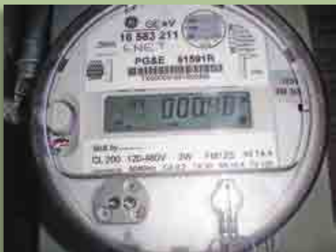
The meter for the Xantrex GT showing net -0.48 KW.
