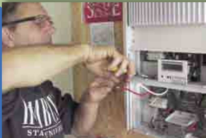
Peter Brant demonstrates how to remove the inverter from its wiring box, a great feature of the Xantrex GT3 series inverters.
