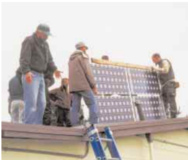
The fun part—puttin' panels on the roof.
